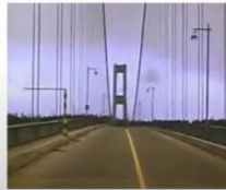
Tacoma Narrows Bridge Collapse
